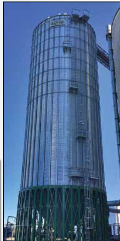
World's Largest Hopper Bin 42' 27 ring - 128,000+ Bushel North Dakota - October 2017
